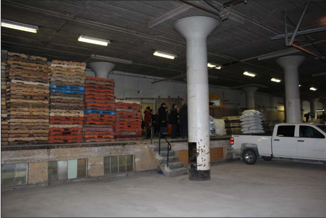
Plate 23 – T. Eaton’s Company Printing Plant & Track Warehouse, 130 Galt Avenue, 1927 building, interior loading dock, 2017. ( M. Peterson, 2017. )
