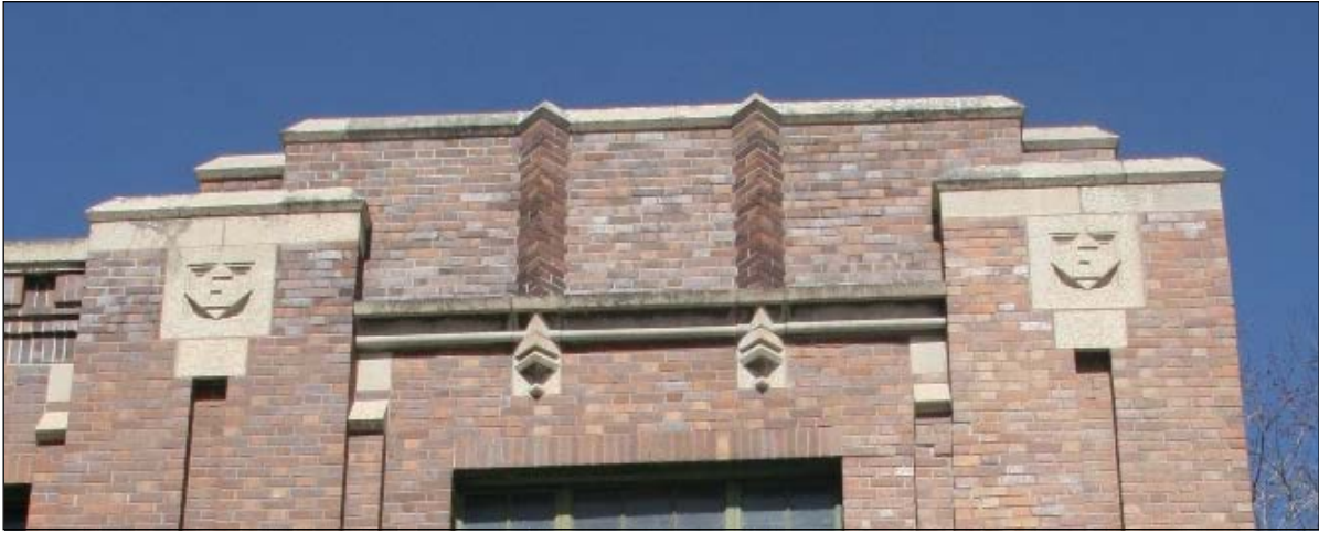
Plate 9 – T. Eaton’s Company Printing Plant & Track Warehouse, 130 Galt Avenue, detail of south façade, 2015. ( M. Peterson, 2015. )
