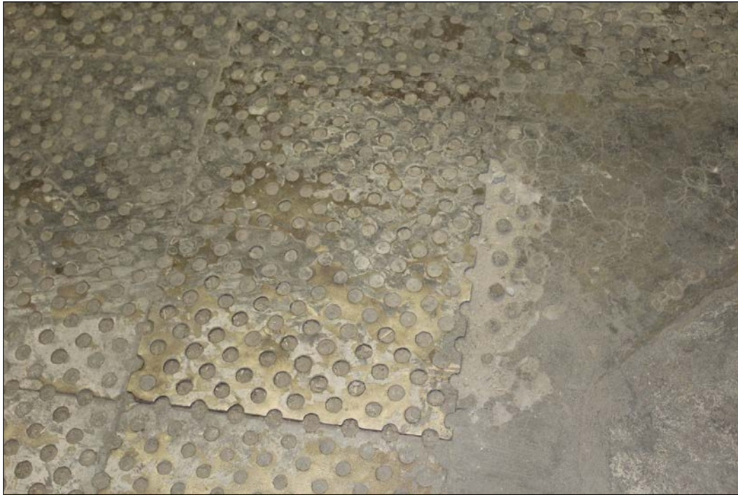
Plate 19 – T. Eaton’s Company Printing Plant & Track Warehouse, 130 Galt Avenue, 1926 building, example of metal cast in concrete for added strength, 2017. ( M. Peterson, 2017. )
