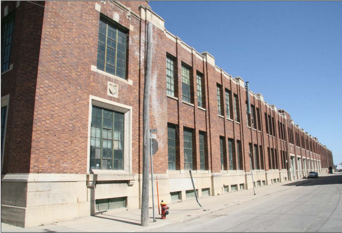
Plate 13 – T. Eaton’s Company Printing Plant & Track Warehouse, 130 Galt Avenue, south façade (west end), 2015. ( M. Peterson, 2015. )
