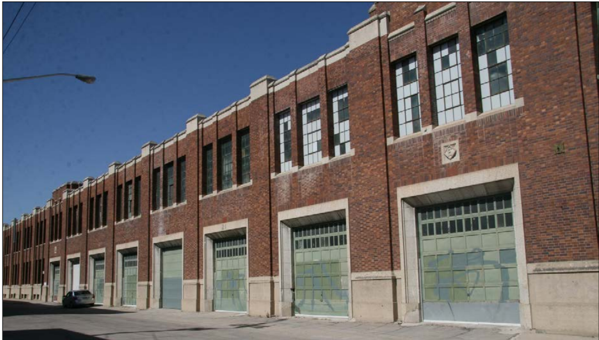
Plate 17 – T. Eaton’s Company Printing Plant & Track Warehouse, 130 Galt Avenue, south side loading doors, 2015. ( M. Peterson, 2015. )
