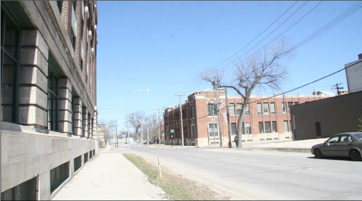
Plate 25 – Lily Street, looking north from Pacific Avenue, 2015. ( M. Peterson, 2015. )
