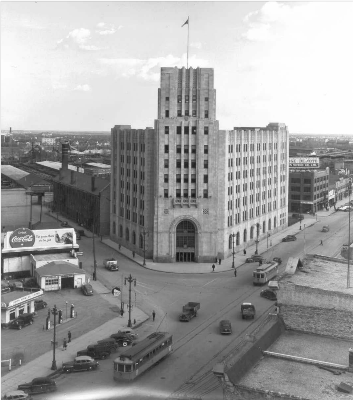
Plate 6 – Federal Building, 269 Main Street, ca.1952. ( M. Peterson Collection. )
