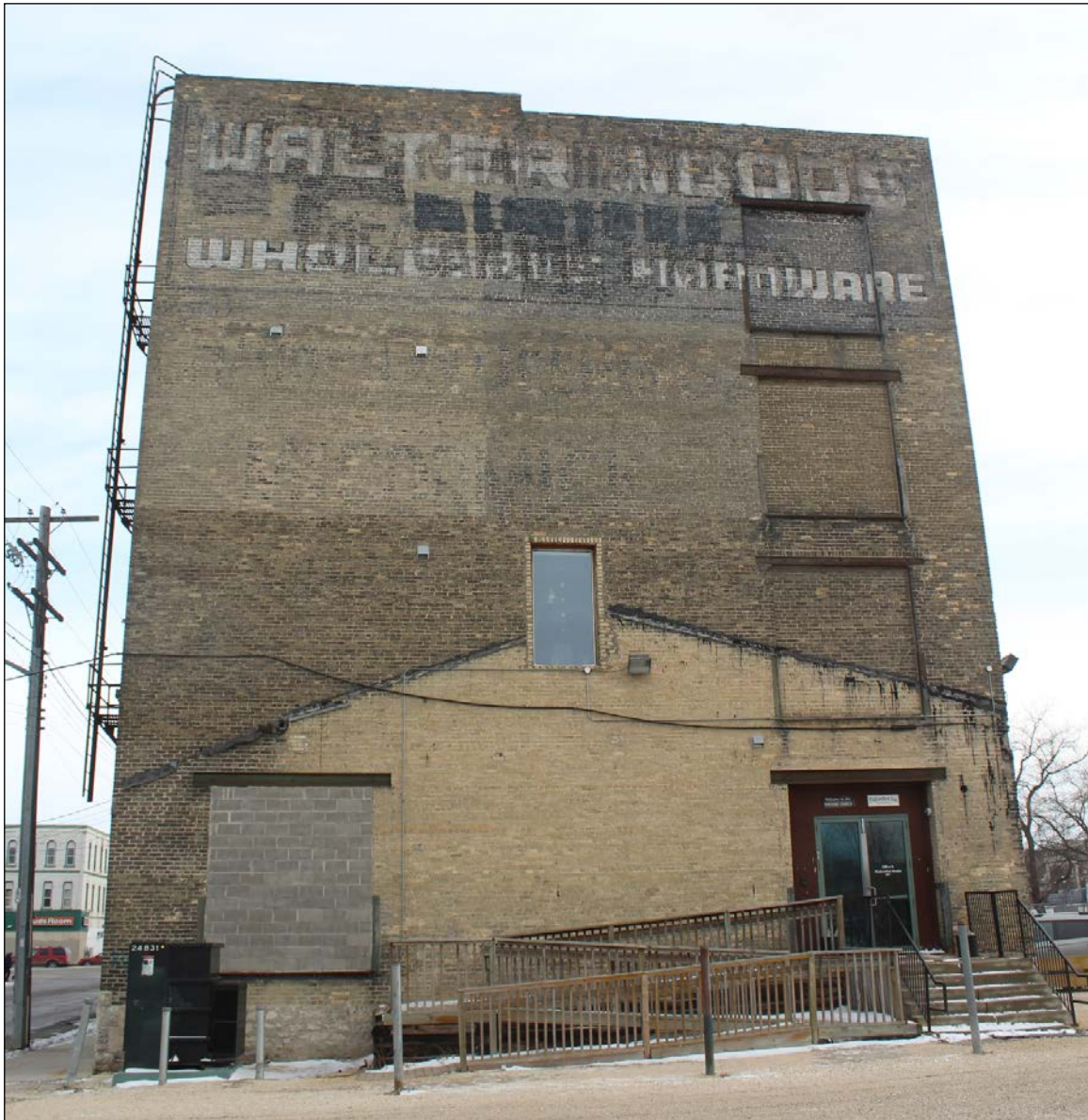
Plate 15 – International Harvester Building, 782 Main Street, rear (west) façade, 2017. ( M. Peterson, 2017. )
