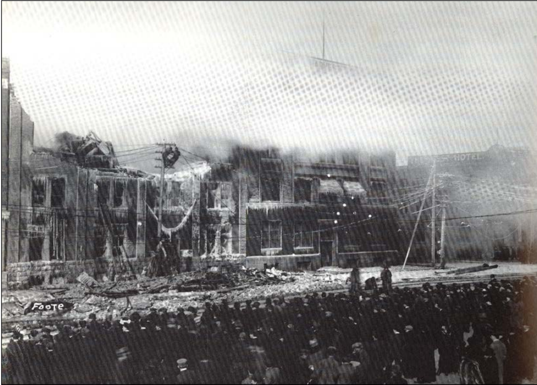
Plate 26 – Aftermath of the March 9, 1912 Radford-Wright Building fire. Partially obscured by the smoke is the International Harvester Building to the right. (Reproduced from V. Leah, Alarm of Fire , [Winnipeg, MB: Firefighters Burn Fund, 1982], p. 64.)
