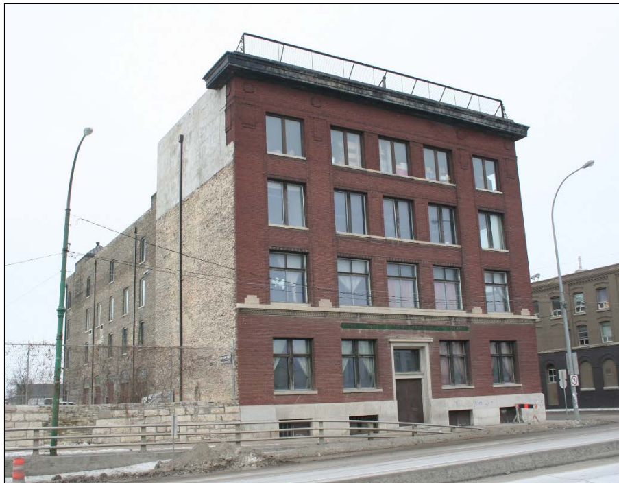
Plate 13 – International Harvester Building, 782 Main Street, front (east) and south façades, 2015. (M. Peterson, 2015.)
