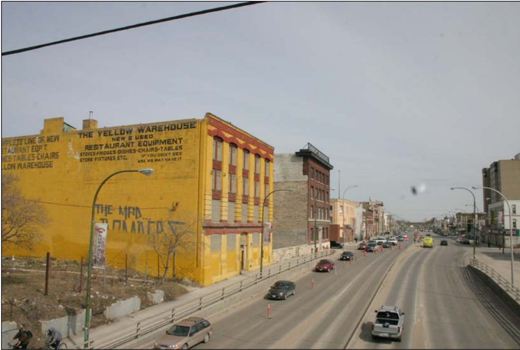
Plate 21 – Main Street looking north from the Higgins Avenue CPR overpass, 2011. The yellow building in the foreground, the Stuart Machinery Warehouse, 764 Main Street (built 1909-1910), was demolished in 2012. (M. Peterson, 2011.)
