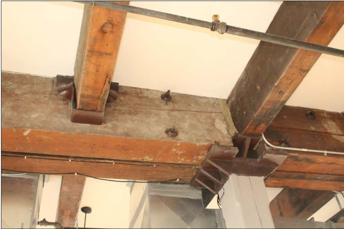
Plate 7 – International Harvester Building, 782 Main Street, example of double beam construction, 2017. ( M. Peterson, 2017. )
