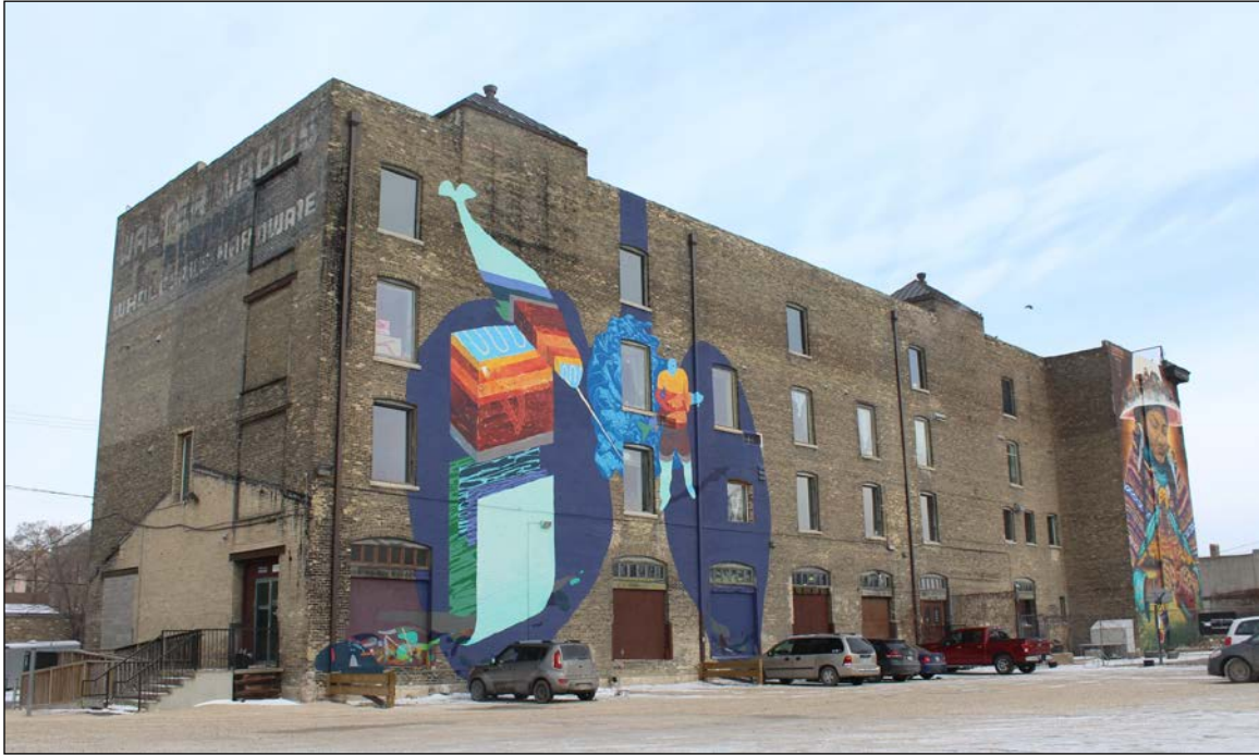
Plate 14 – International Harvester Building, 782 Main Street, rear (west) and south façades, 2017. (M. Peterson, 2017.)
