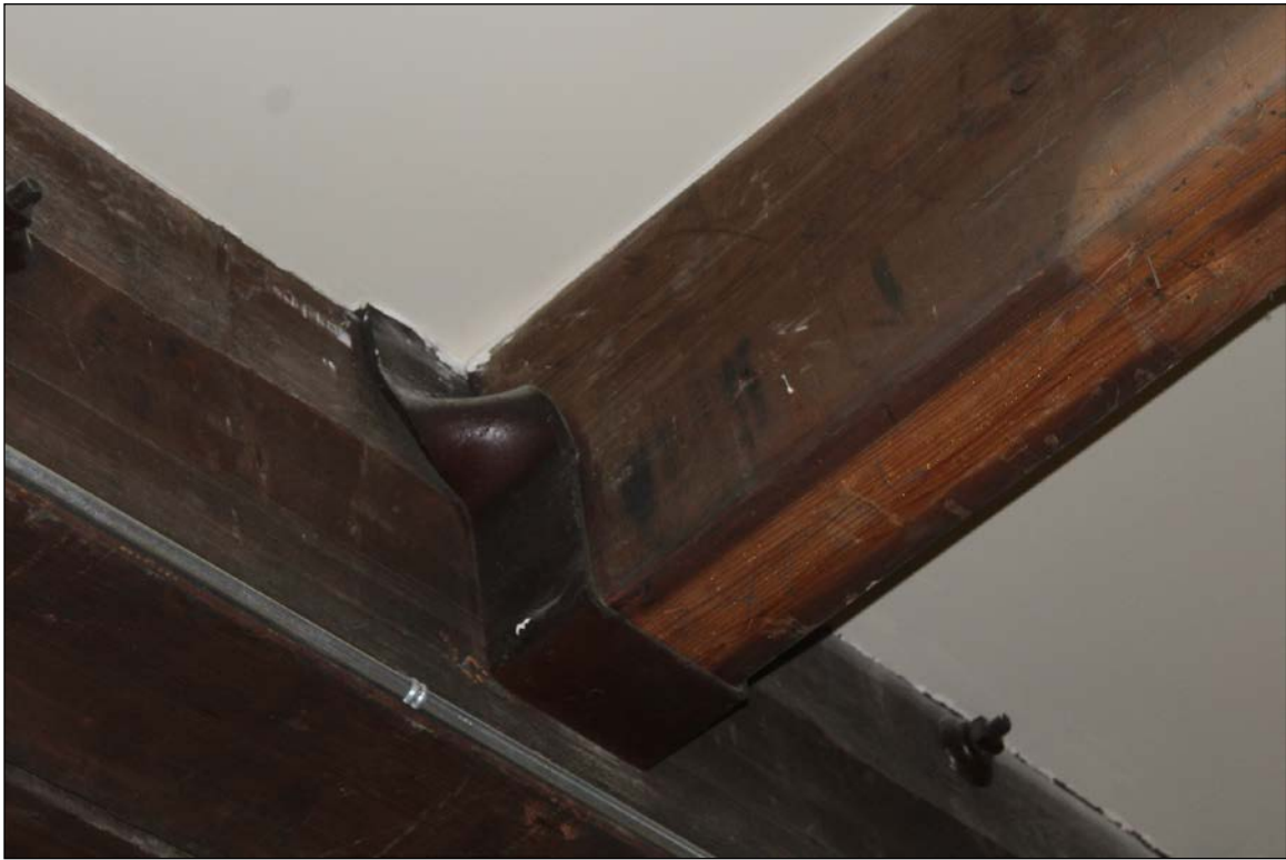
Plate 8 – International Harvester Building, 782 Main Street, example of ornate, curved beam hanger, 2017. ( M. Peterson, 2017. )
