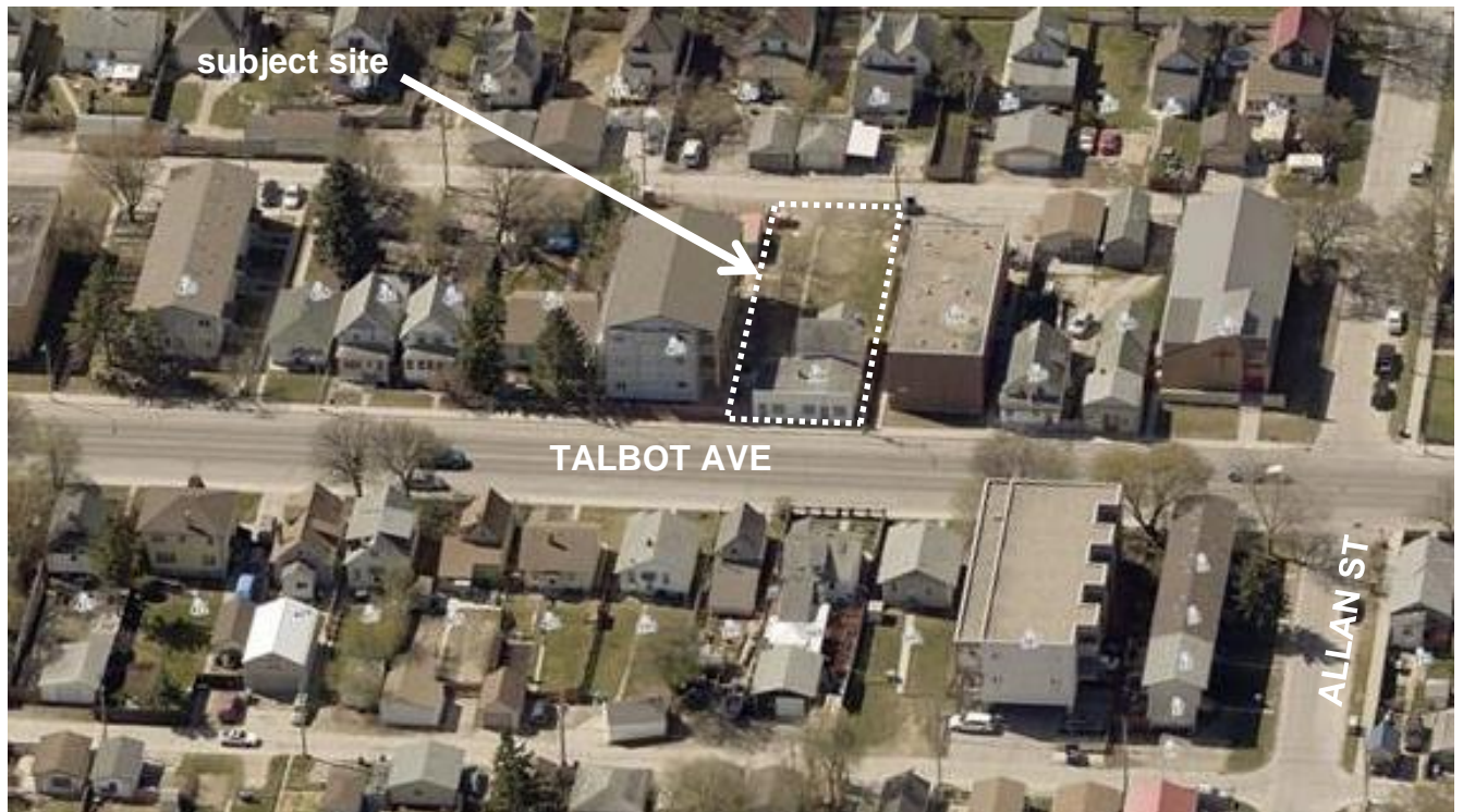
Figure 1: Looking South, image derived from 2018 aerial photography
