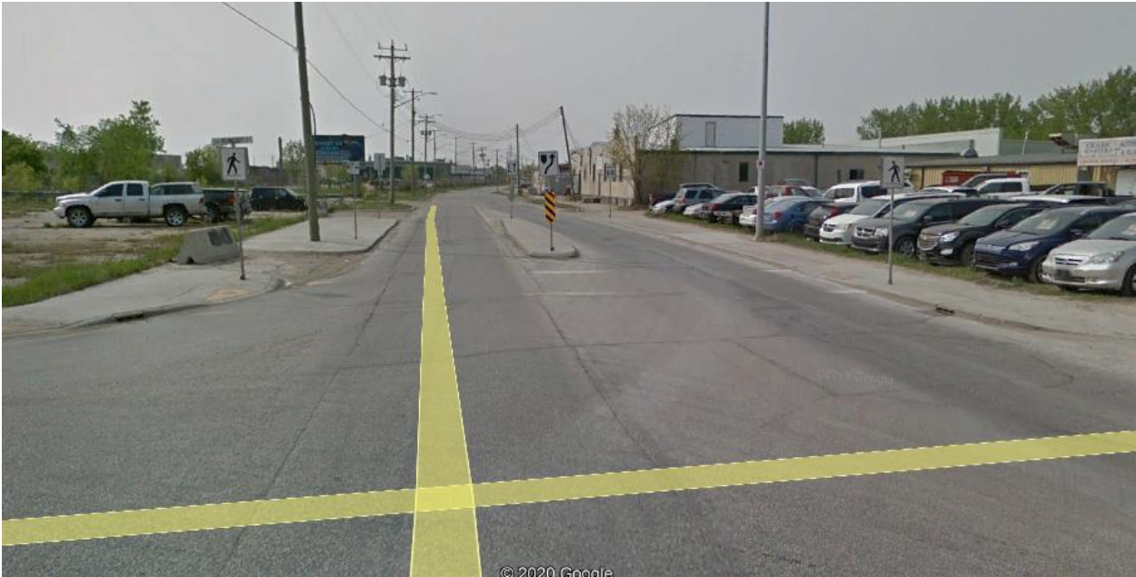
Figure 2: Pedestrian Crosswalk on Archibald Street at Plinguet Street (facing southbound)
