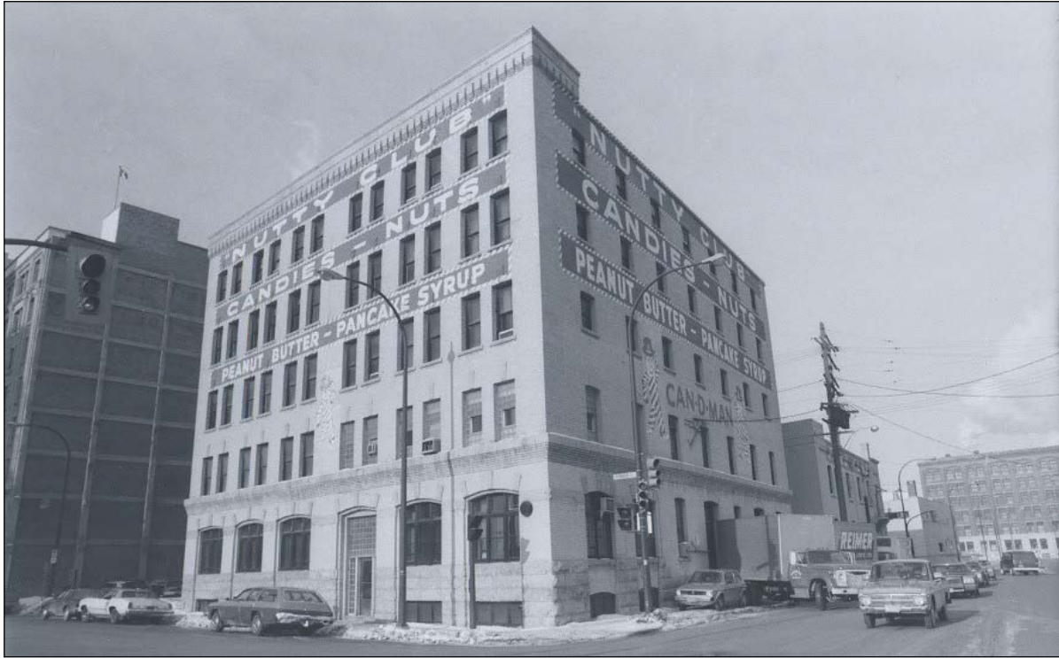
Plate 18 – Scott-Bathgate Building, 149 Pioneer Avenue, 1978. ( City of Winnipeg. )
