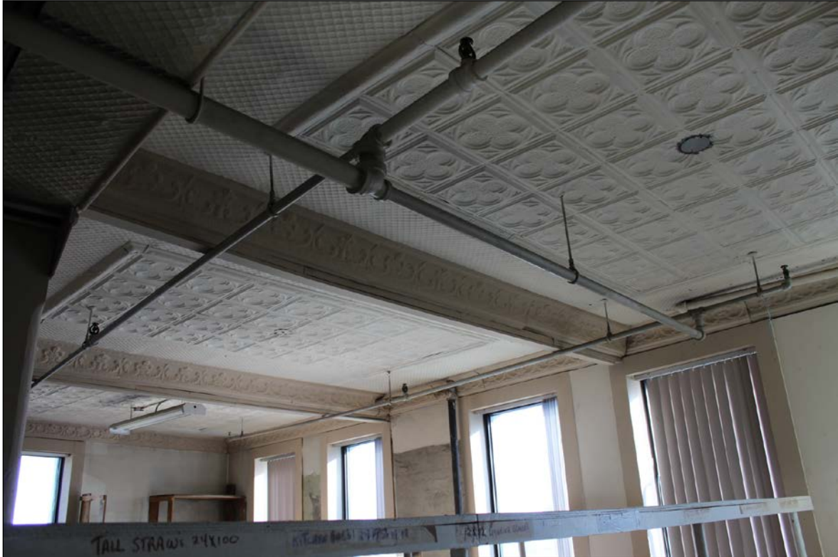
Plate 12 – Scott-Bathgate Building, 149 Pioneer Avenue, 3 rd floor ornamental tin ceiling in original office/sample room area, 2017. ( M. Peterson, 2017. )
