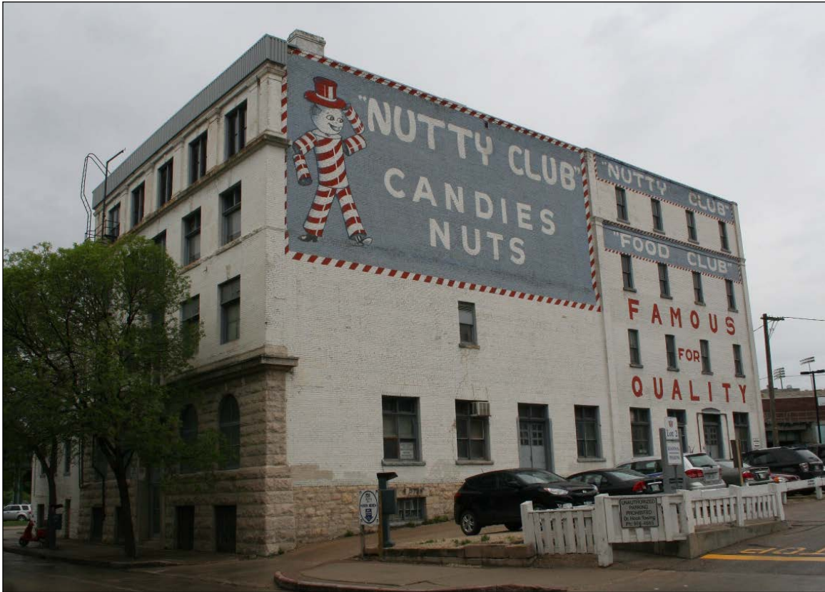
Plate 23 – Thomas Black Building, 80 Lombard Avenue, 2014. Built in stages between 1896 and 1907, the structure was taken over by Scott-Bathgate Company ca.1945. ( M. Peterson, 2014. )
