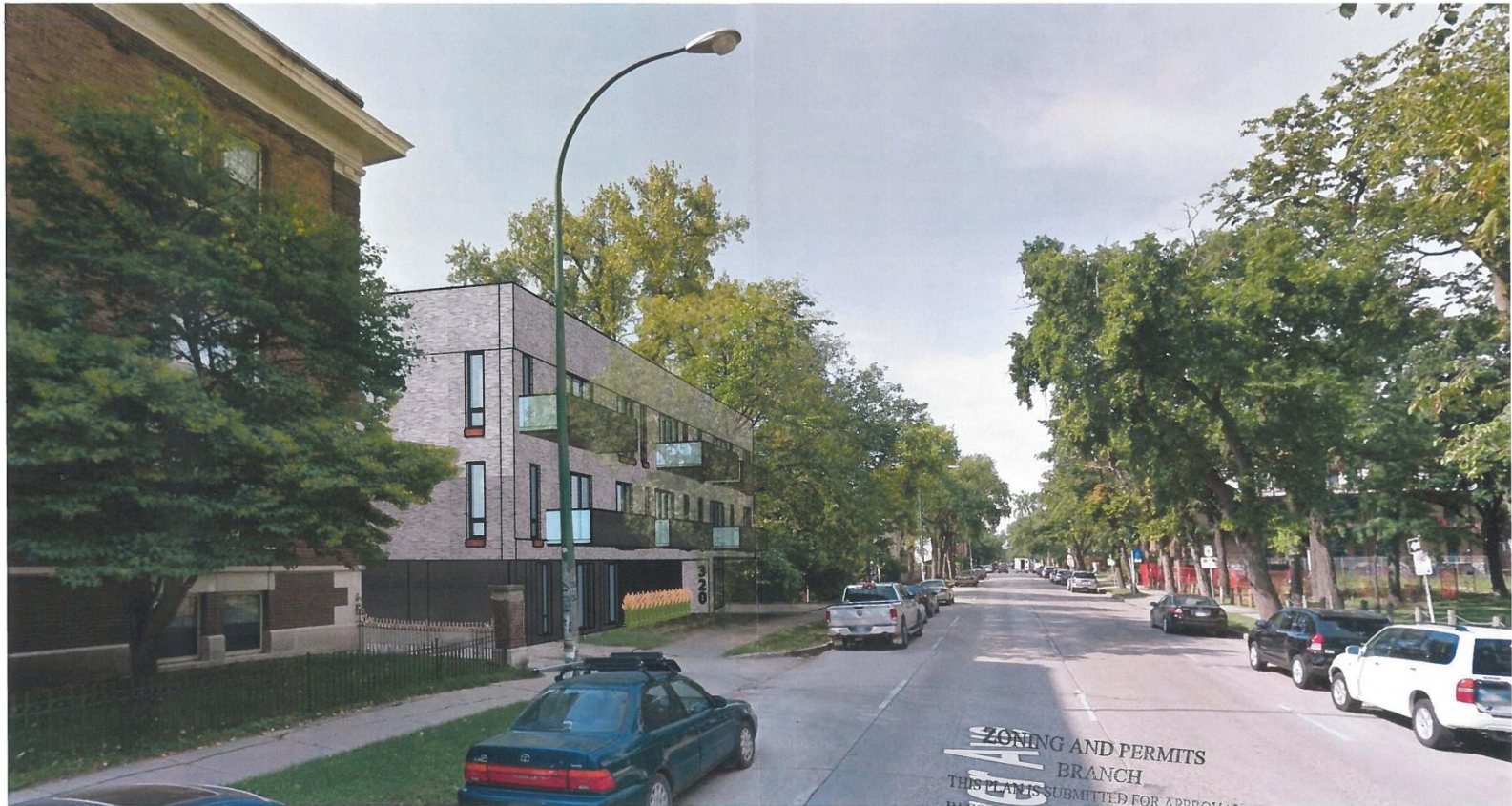
NORTH-EAST ELEVATION - LOOKING WEST DOWN RIVER AVE.
