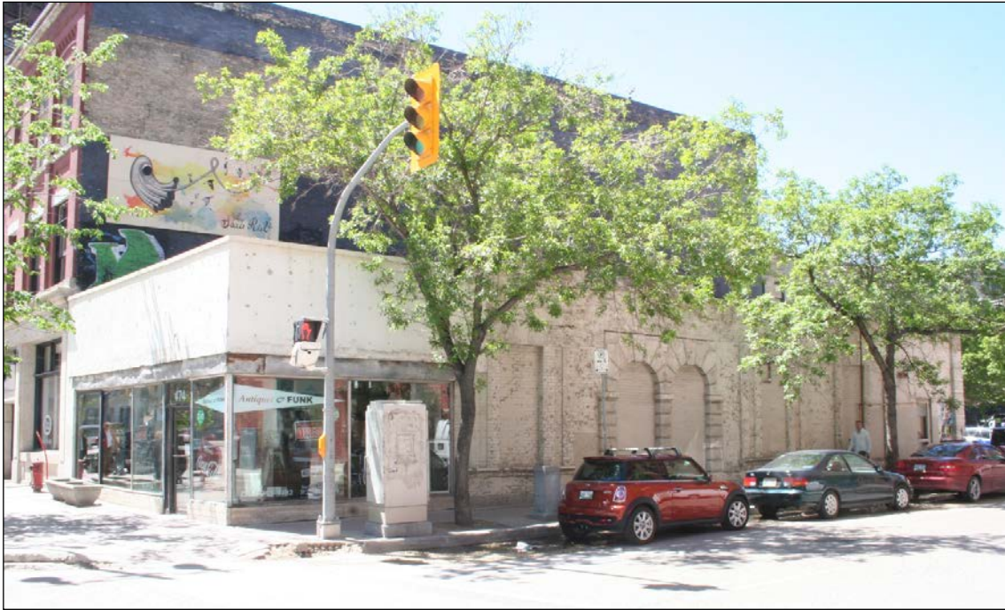
Plate 6 – Duffin Block, 474 Main Street, front (east) and north façades, 2014. ( M. Peterson, 2014. )
