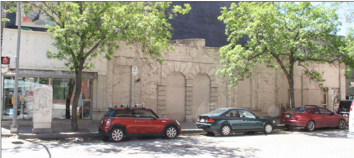
Plate 11 – Duffin Block, 474 Main Street, north façade, 2014. (M. Peterson, 2014.)
