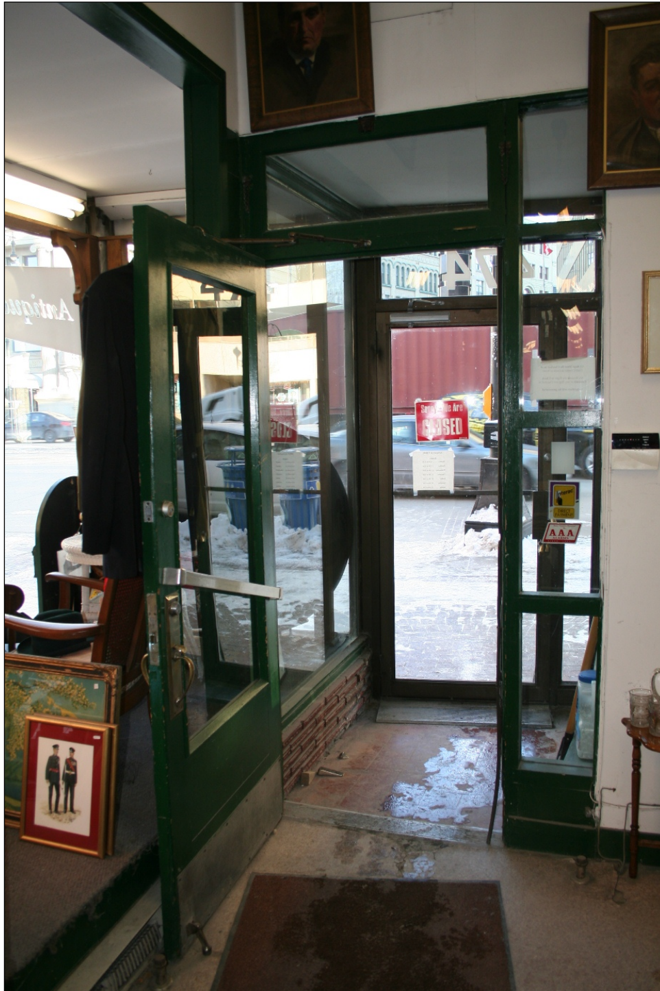
Plate 16 – Duffin Block, 474 Main Street, front entrance foyer, 2014. (M. Peterson, 2014.)
