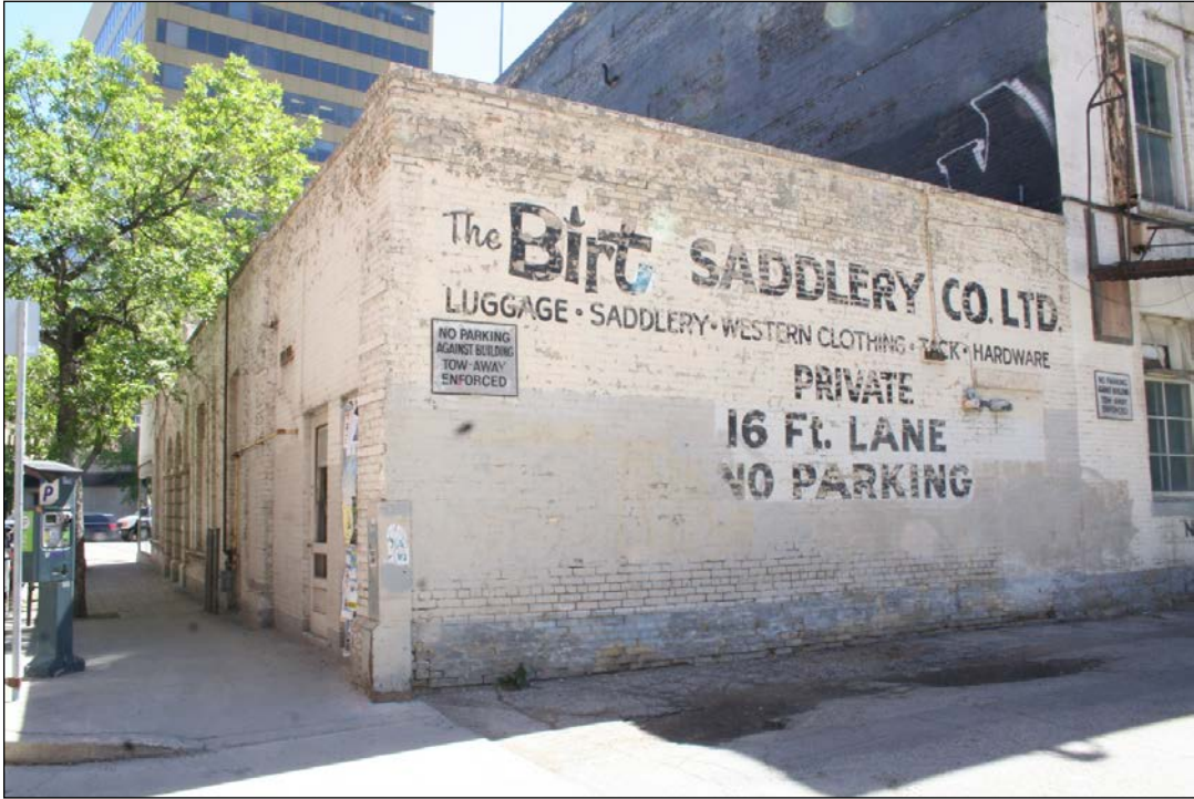
Plate 14 – Duffin Block, 474 Main Street, rear (west) façade, 2014. ( M. Peterson, 2014. )
