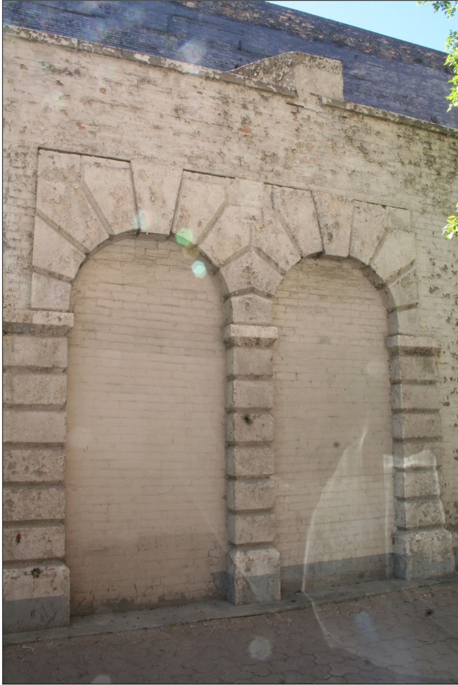
Plate 12 – Duffin Block, 474 Main Street, detail of north façade, 2014. (M. Peterson, 2014.)
