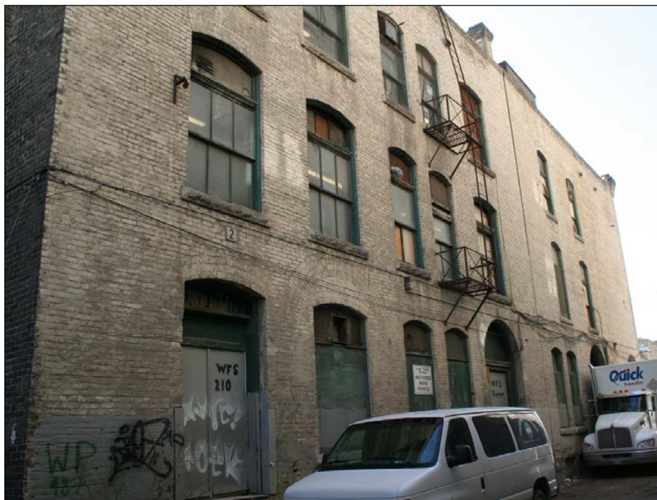
Plate 12 – McLaughlin Carriage Company Building, 208 Princess Street, rear (west) façade, 2015. (M. Peterson, 2015.)
