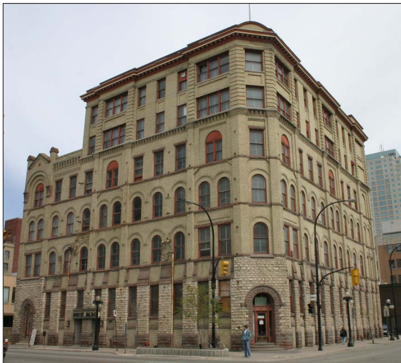
Plate 6 – 33 Princess Street, Peck Building, built 1893, C.H. Wheeler, architect. ( City of Winnipeg, 2005. )
