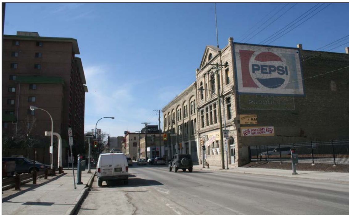
Plate 18 –Princess Street looking south, 2015. ( M. Peterson, 2015. )
