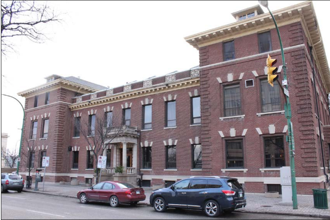
Plate 13 – Manitoba Club, 194 Broadway, front (north) façade, 2016. (M. Peterson, 2016.)
