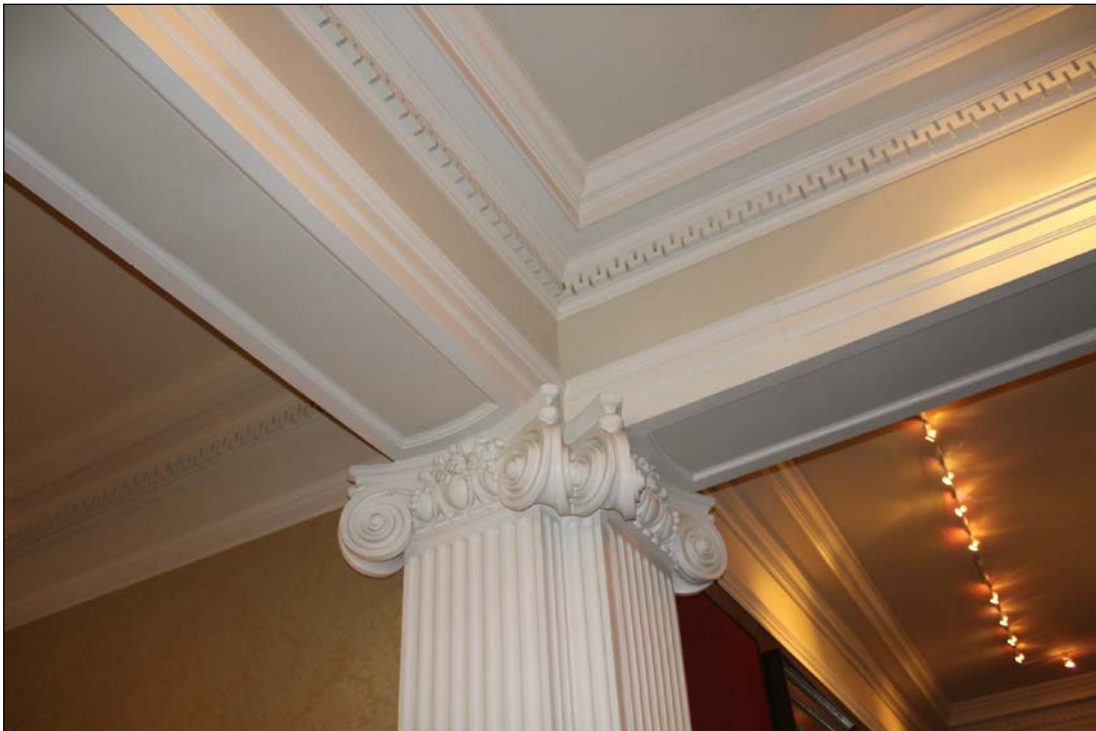
Plate 29 – Manitoba Club, 194 Broadway, second floor, hallway detail, 2017. ( M. Peterson, 2017. )
