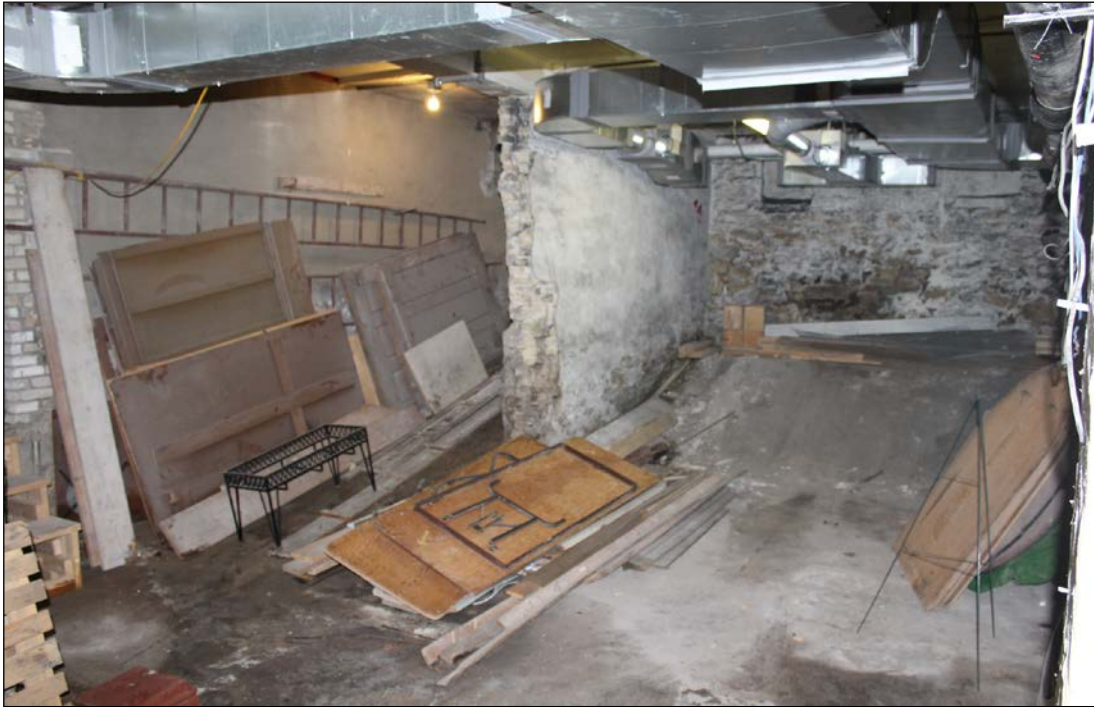
Plate 22 – Manitoba Club, 194 Broadway, basement, former boiler and coal room, 2017. ( M. Peterson, 2017. )
